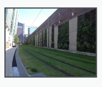
The bed of tram lines can be greened to improve amenity and reduce the rate of surface runoff, such as this grassed tramway at Birmingham Snow Hill station
